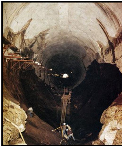
Fig. 4.5 Cavitation in spillway of Glen Canyon Dam [8]
