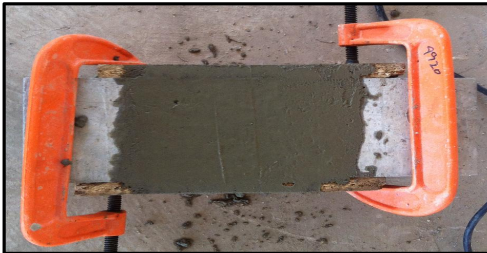
Fig. 3.3 A PCC repaired Column with formwork
