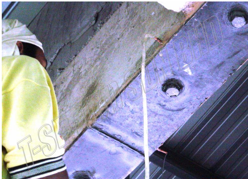
Figure 2.3: Steel plate bonding
