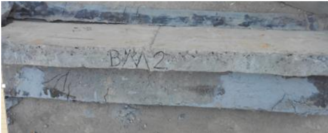
Figure 3.7: Failure pattern of BEAM2
