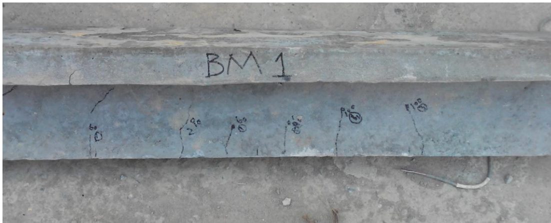
Figure 3.6: Failure pattern of BEAM1
