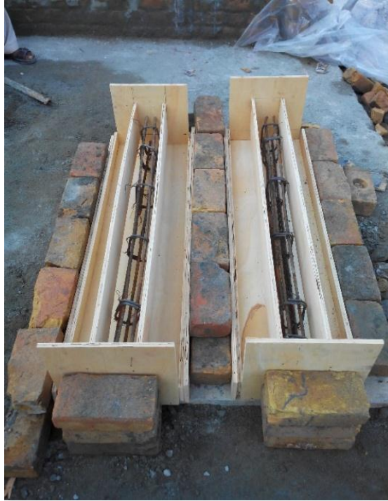
Figure 3.1: Formwork and cage of reinforcement
