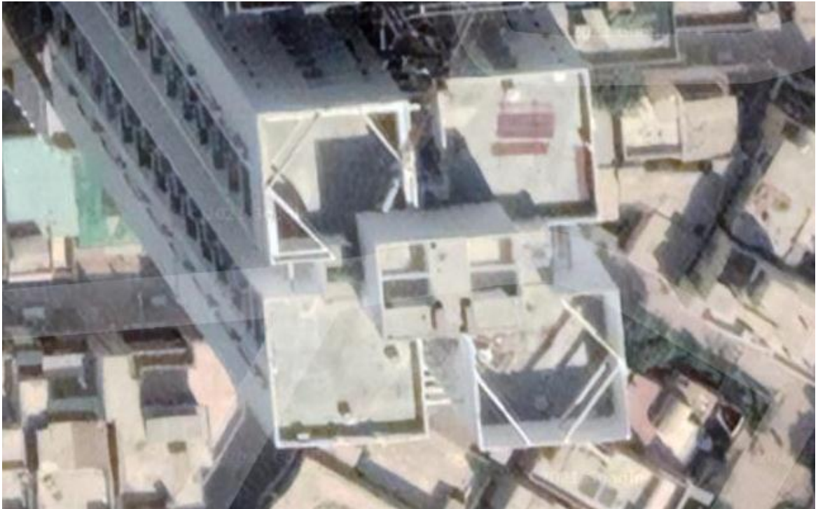
Figure 10 Aerial view of Lucky Mall Apartments Tower A depicting current condition
