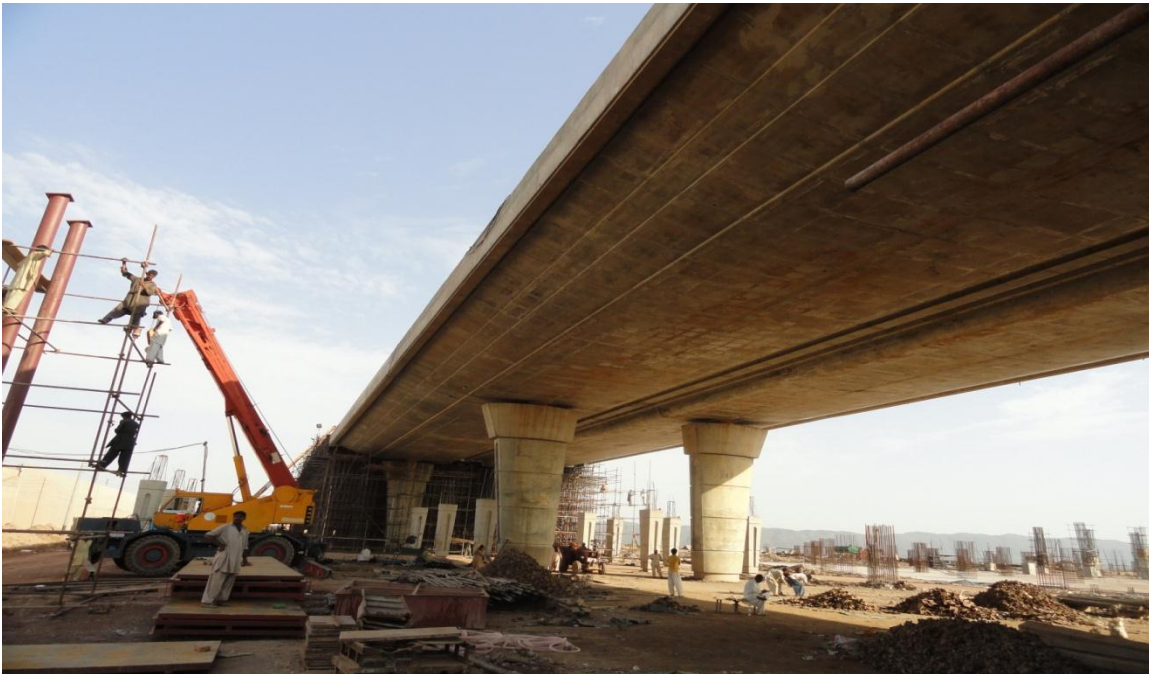
Figure 8: Departure level bridge under construction
