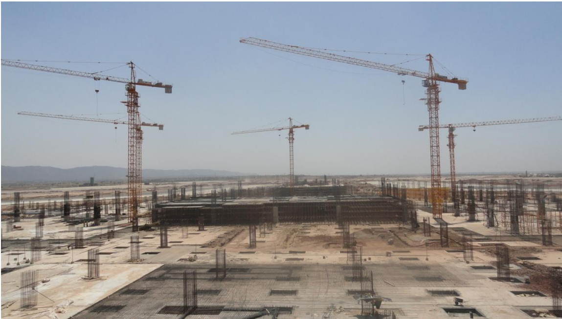
Figure: 11 Construction of foundations of the Passenger Terminal building
