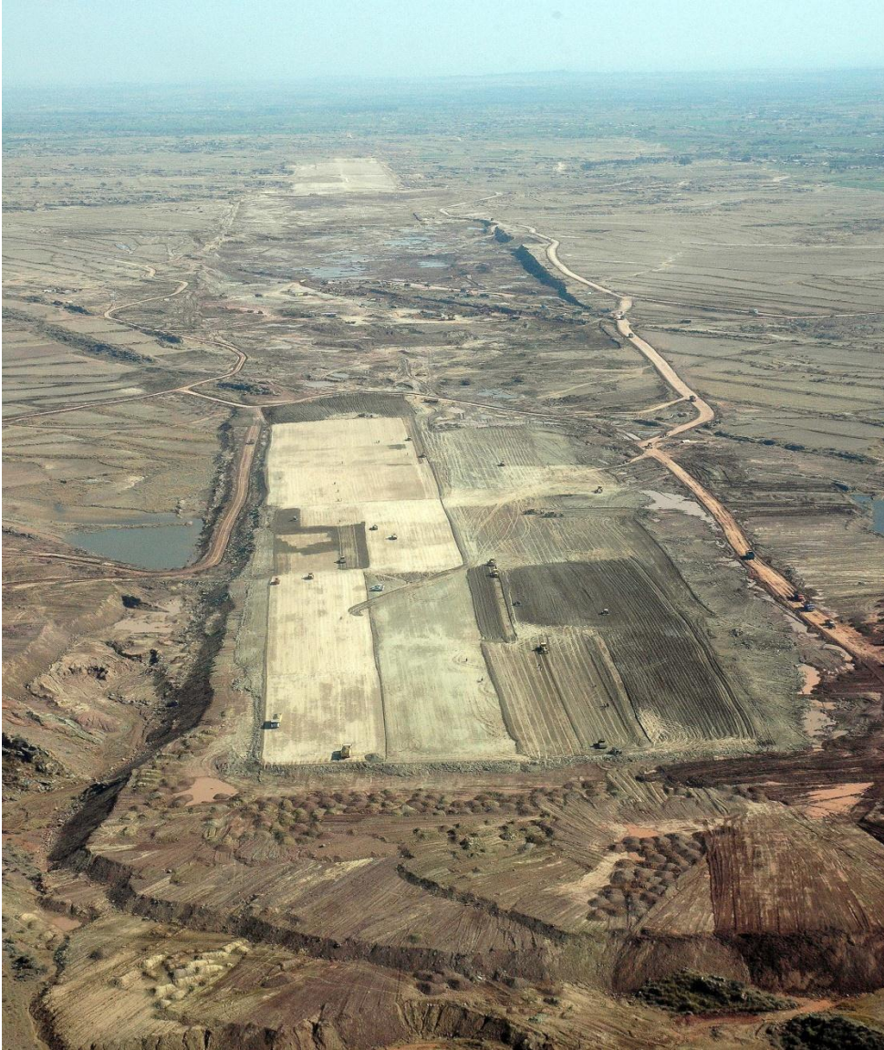
Figure 5: Package 1 (airside infrastructure) Land clearing for runways
