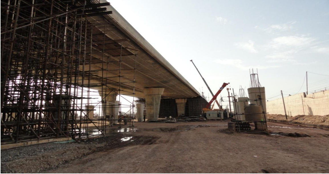
Figure 9: Another view of Departure level bridge under construction
