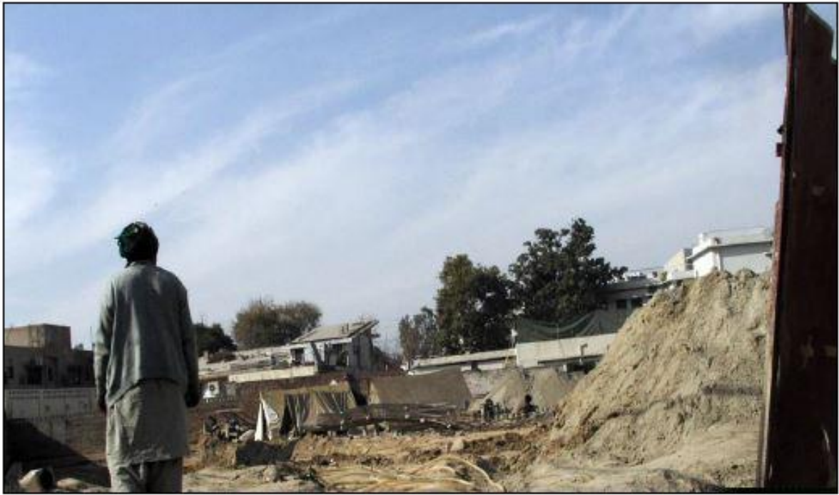
Figure 15: An overview of adjacent buildings on rear end of building
