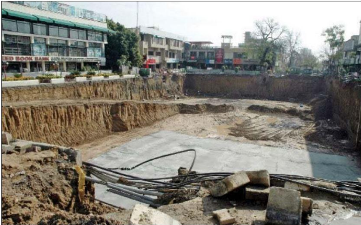
Figure 13: Excavation for southern parking plaza Jinnah Super Market F-7, Islamabad
