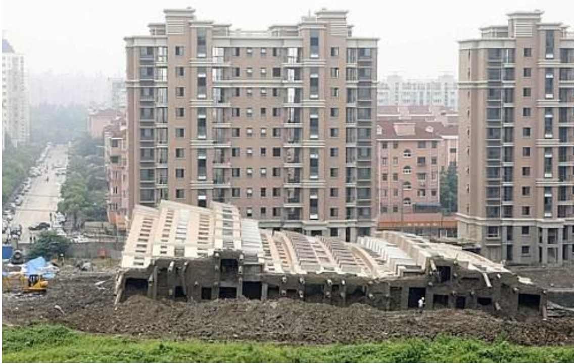
Figure 1: Shanghai 13-storey block of flats collapsed on 28 th June 2009 due to piling under building for a car parking (The Wall Street Journal 2009)
