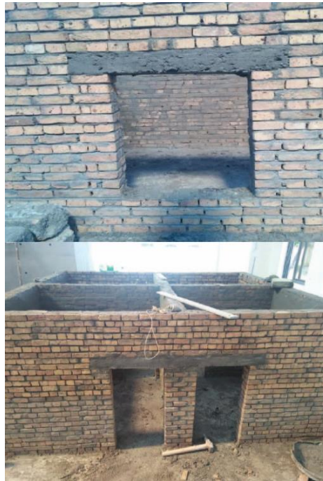
Figure 26 Model in Construction Phase
