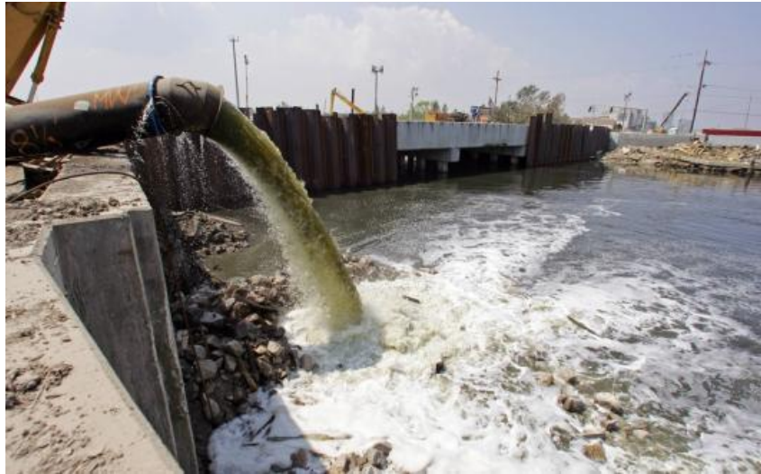
Figure 3.3: Discharge of tanneries wastewater at Kasur tannery treatment plant
