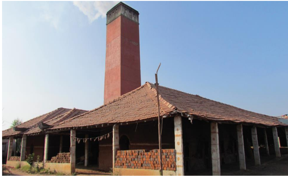
Figure 2-6: A typical view of down draught kiln [16]
