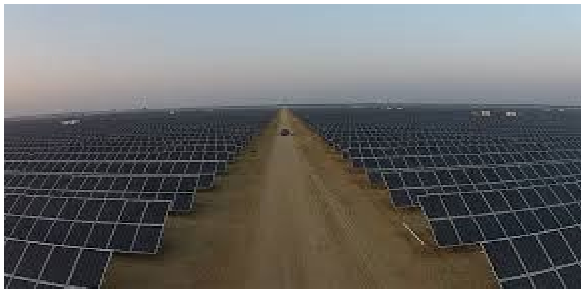
Figure 2.2 PV Power Plant [70]
