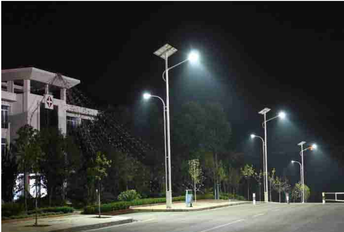
Figure 2.1 PV Road Lights [65]
