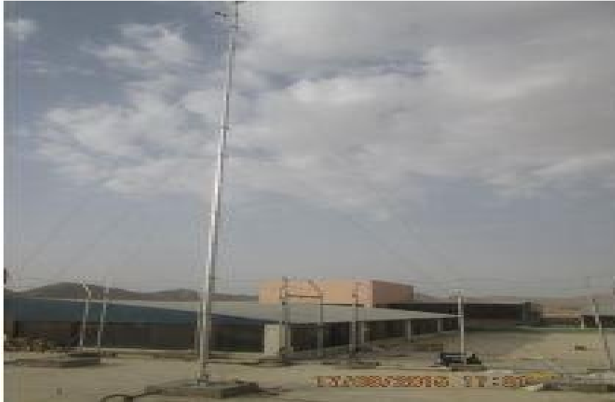
Figure 3.3 Device Installed at BUITEMS Quetta
