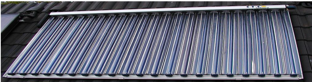
Figure 2-3: Evacuated Plate solar collector
