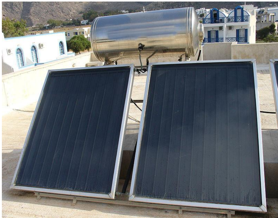
Figure 2-2: Flat plate thermal system for water heating
