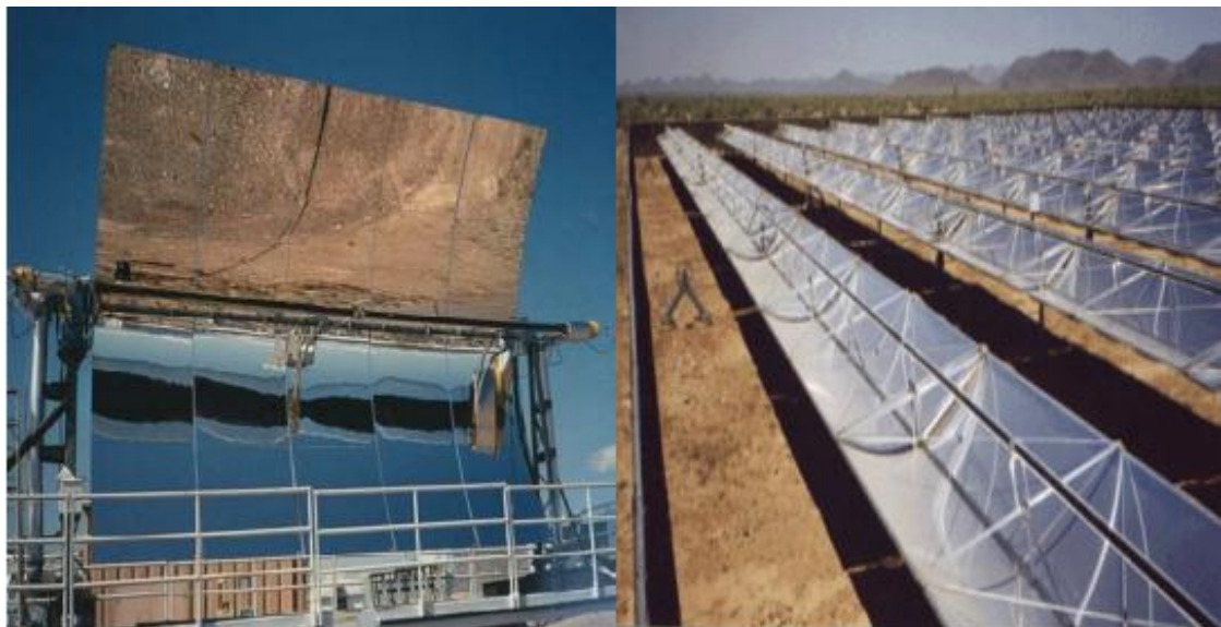
(c) Parabolic trough collectors
