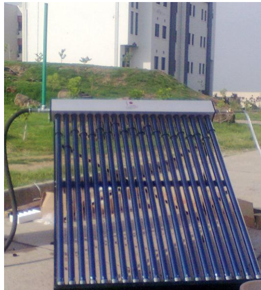
Figure 4.2: Heat pipe evacuated tube solar thermal manipulate
