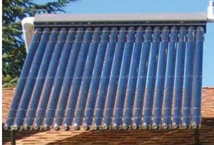
Figure 2.13: Evacuated tube collector [24]
