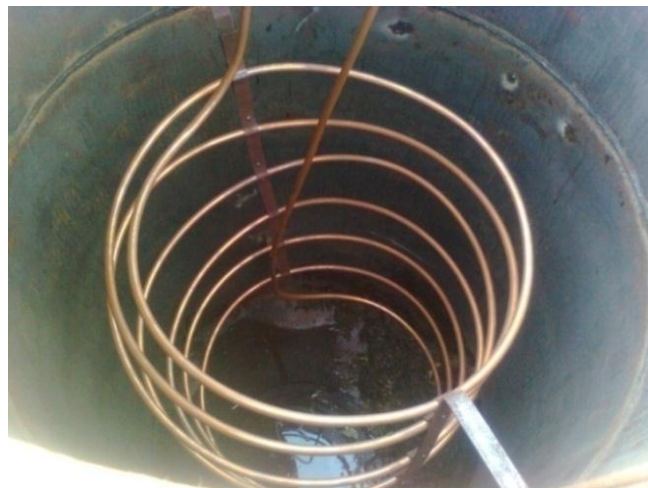
Figure 3.2: Cross sectional area of biogas plant showing copper coils for hot water circulation
