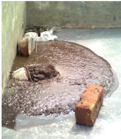
Figure 4.9: Effluent slurry from biogas plant collected in the effluent tank
