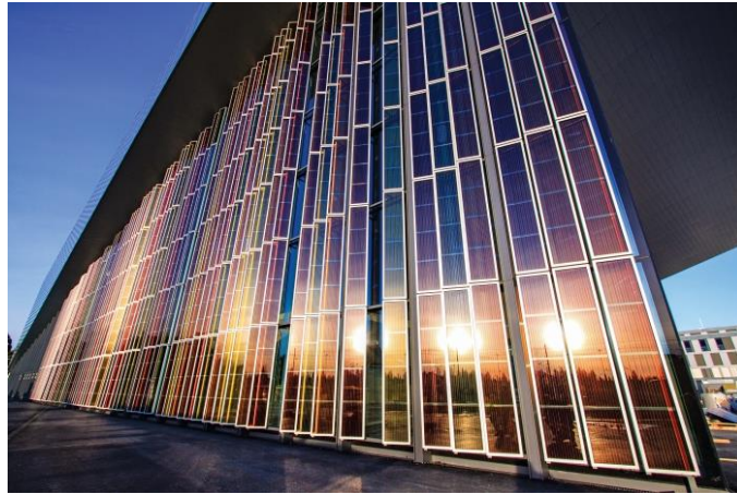
Figure 1-10: Dye-sensitized solar cells integrated SwissTech Convention Center made by Soloronix [27].
