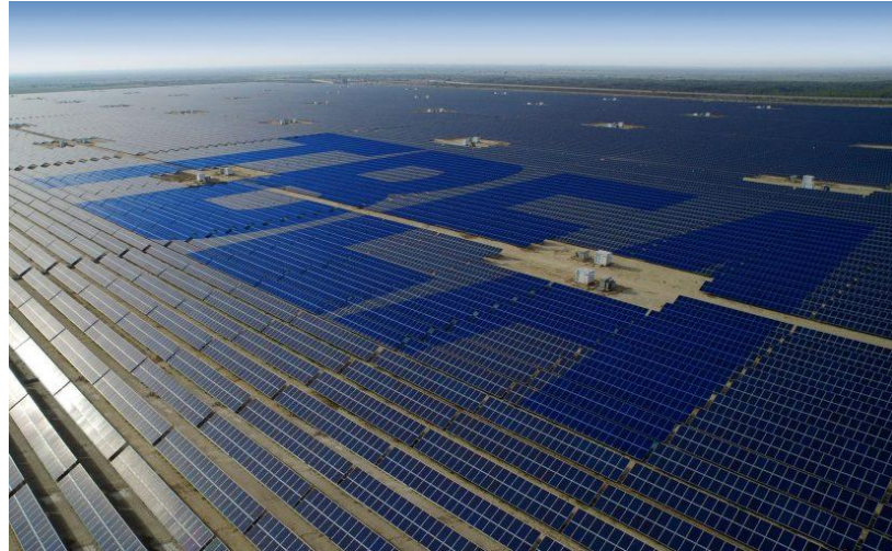
Figure 1-1: Quaid-e-Azam Solar Park with a capacity of 1,000 MW [17].
