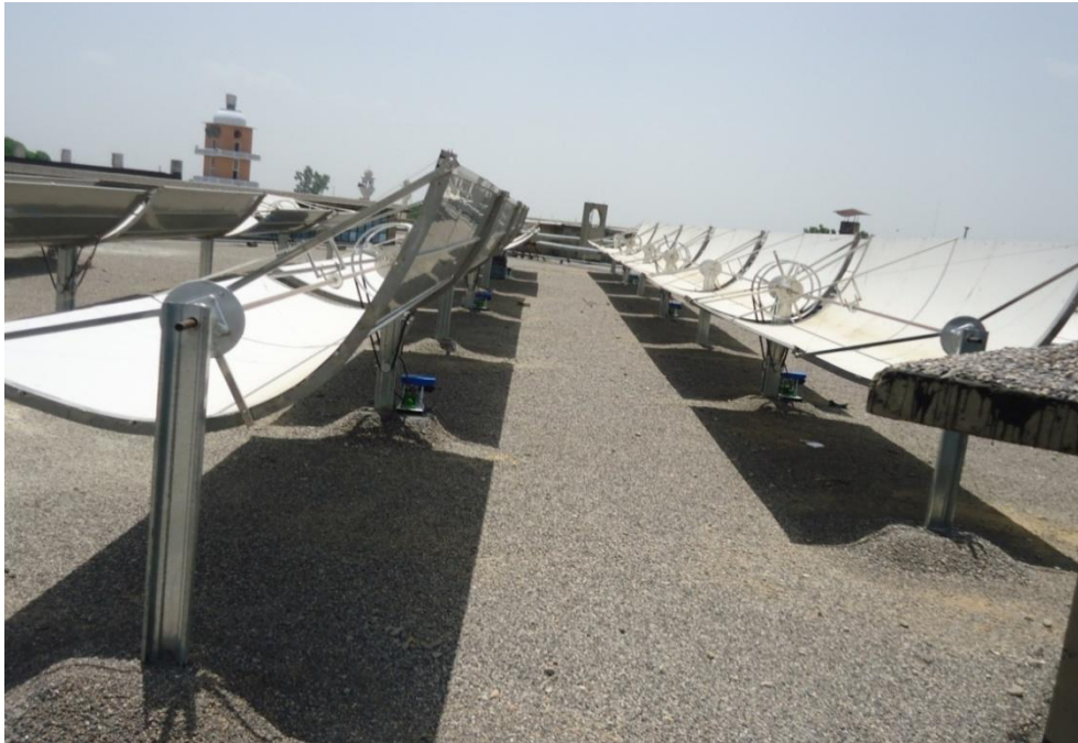
Fig. 4. 8 The specific spacing between back to back trough to avoid shadow
