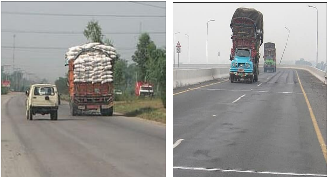
Figure 2.2: Causes of deterioration – Overloading
