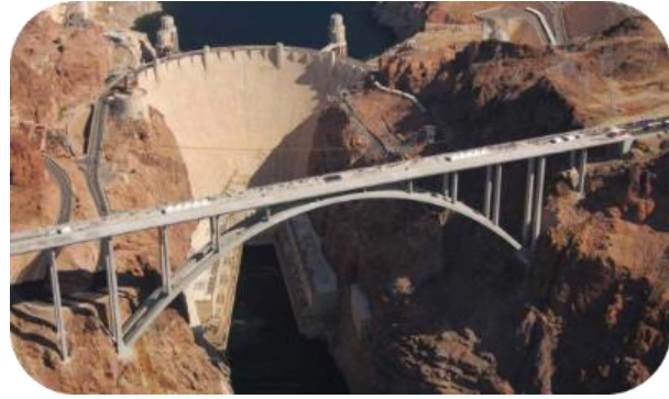
b) Fast Track Construction of a Bridge
