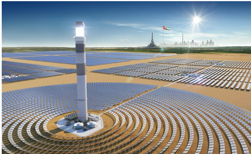
Figure 1-3 Concentrated solar power plant [13]
