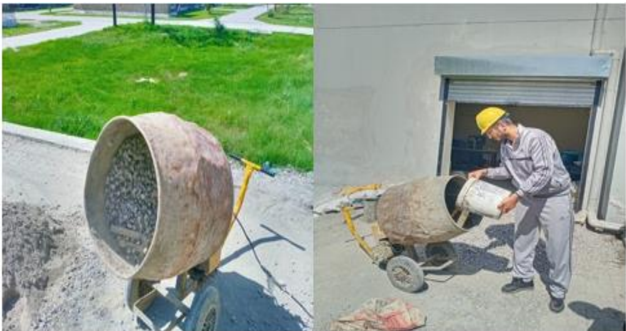
Figure 3.6 Mixing of Concrete
