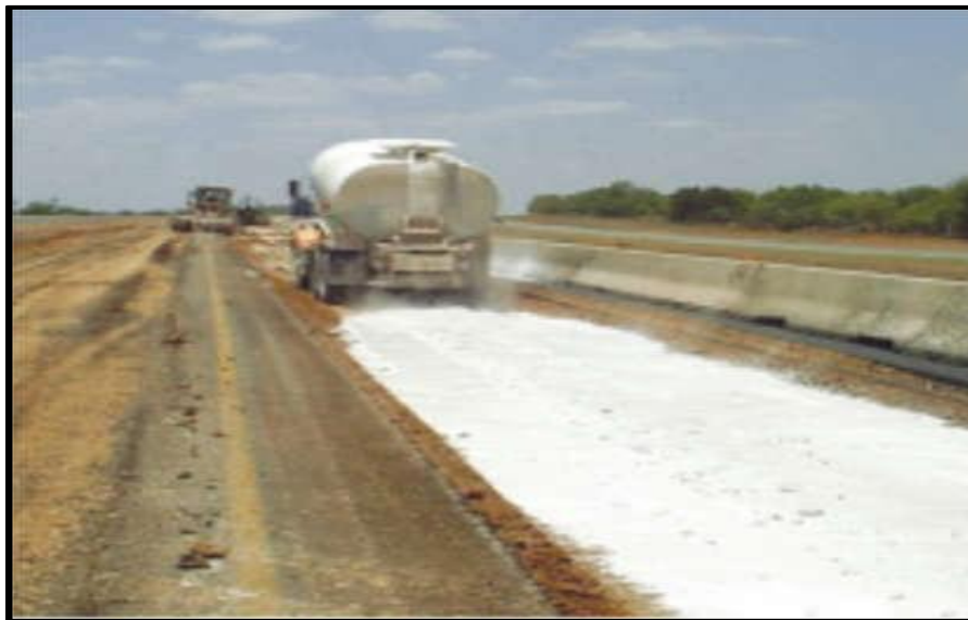
Figure 1-1 Application of Lime on Subgrade
