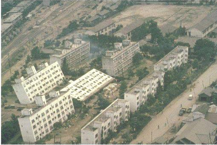
Figure 1.1 Soil Liquefaction, June 16, 1964 Niigata Japan
