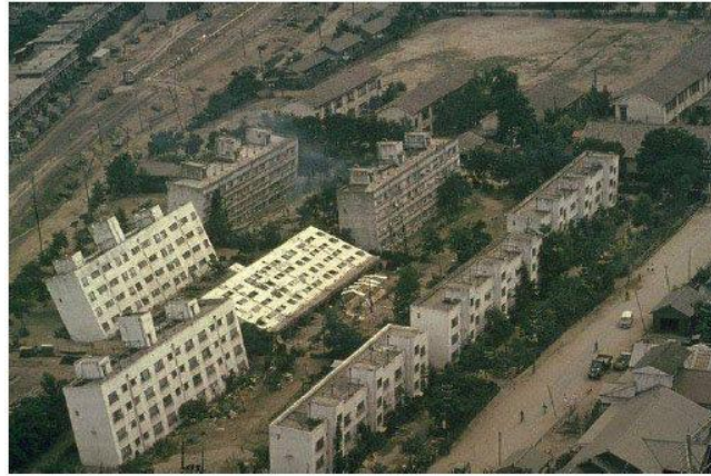
Figure 14.1 Tilted Apartment buildings in Kawagishi Cho, Japan, 1964
