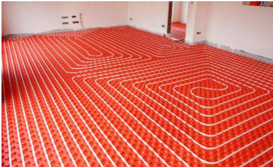
Figure. 3. 8 Radiant floor scheme for space heating
