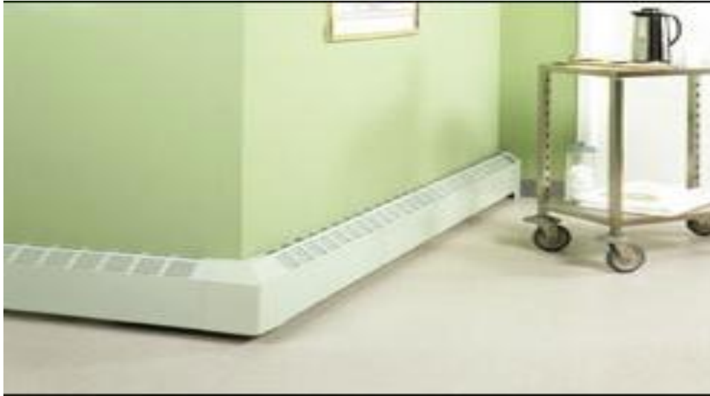
Figure. 3. 7 Base board units for space Heating Scheme
