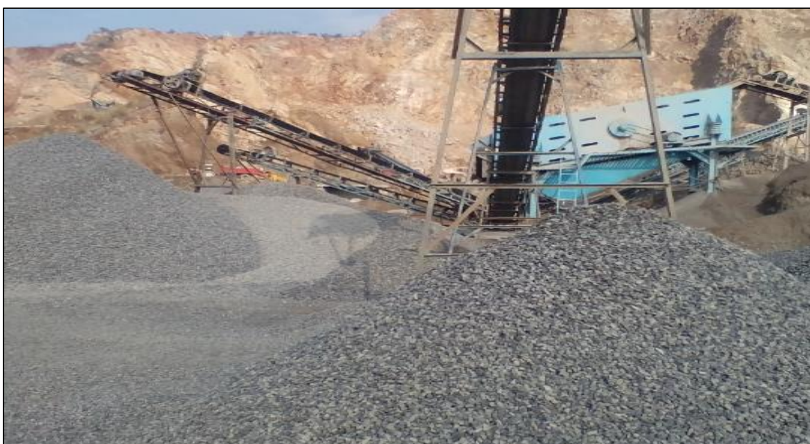
Figure 3.2 Babuzai Quarry Site
