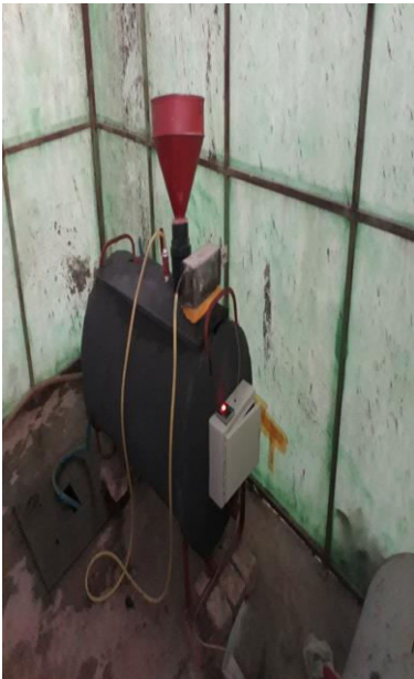
Figure 24 Reactor after construction
