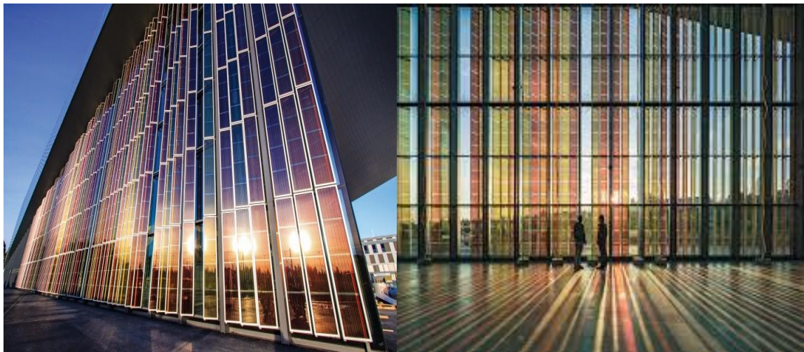
Figure 1-8 Application of building integrated dye-sensitized solar cells
