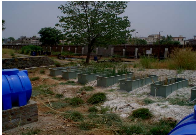
Figure 3.3. The wastewater application to into constructed wetlands for treatment.
