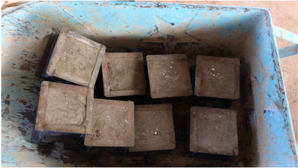
Figure 8: Concrete Blocks to be De-molded
