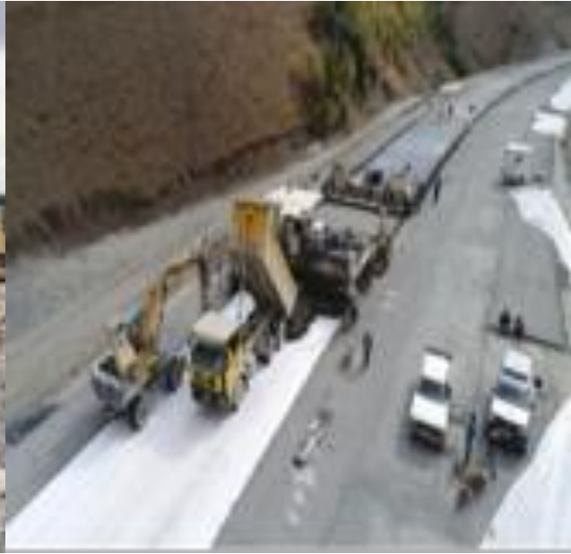
(b)Applications of non-woven geotextiles on Roads
