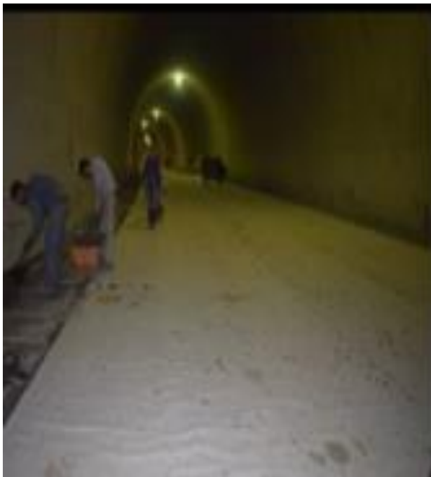
(c) Applications of non-woven geotextiles on tunnel Roads
