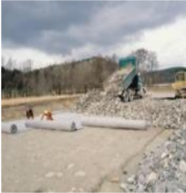
(a)Applications of non-woven geotextiles on Roads
