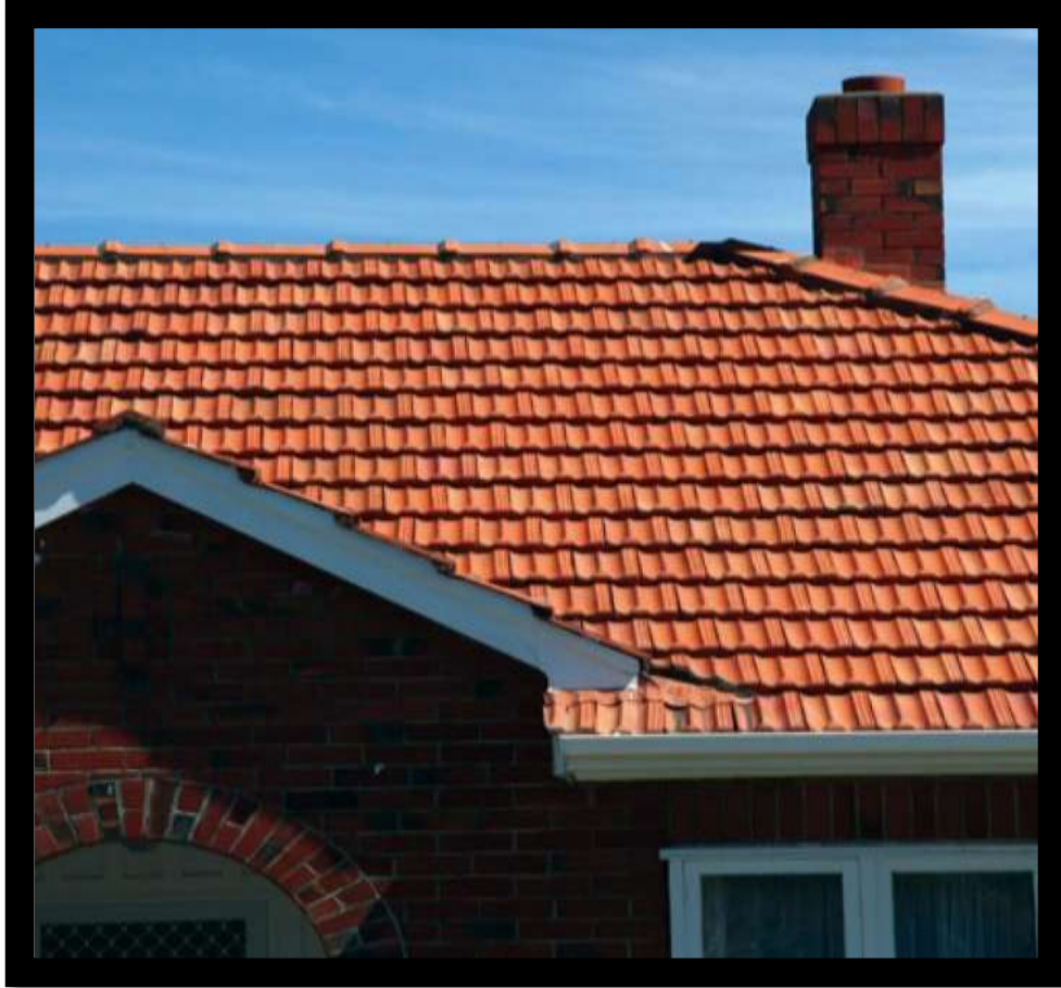
Figure 27: Cladding tiles on roof
