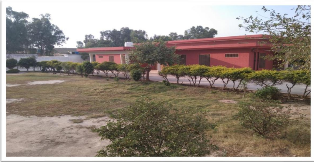
Figure 4-5 Community Center in Old Labor Colony
