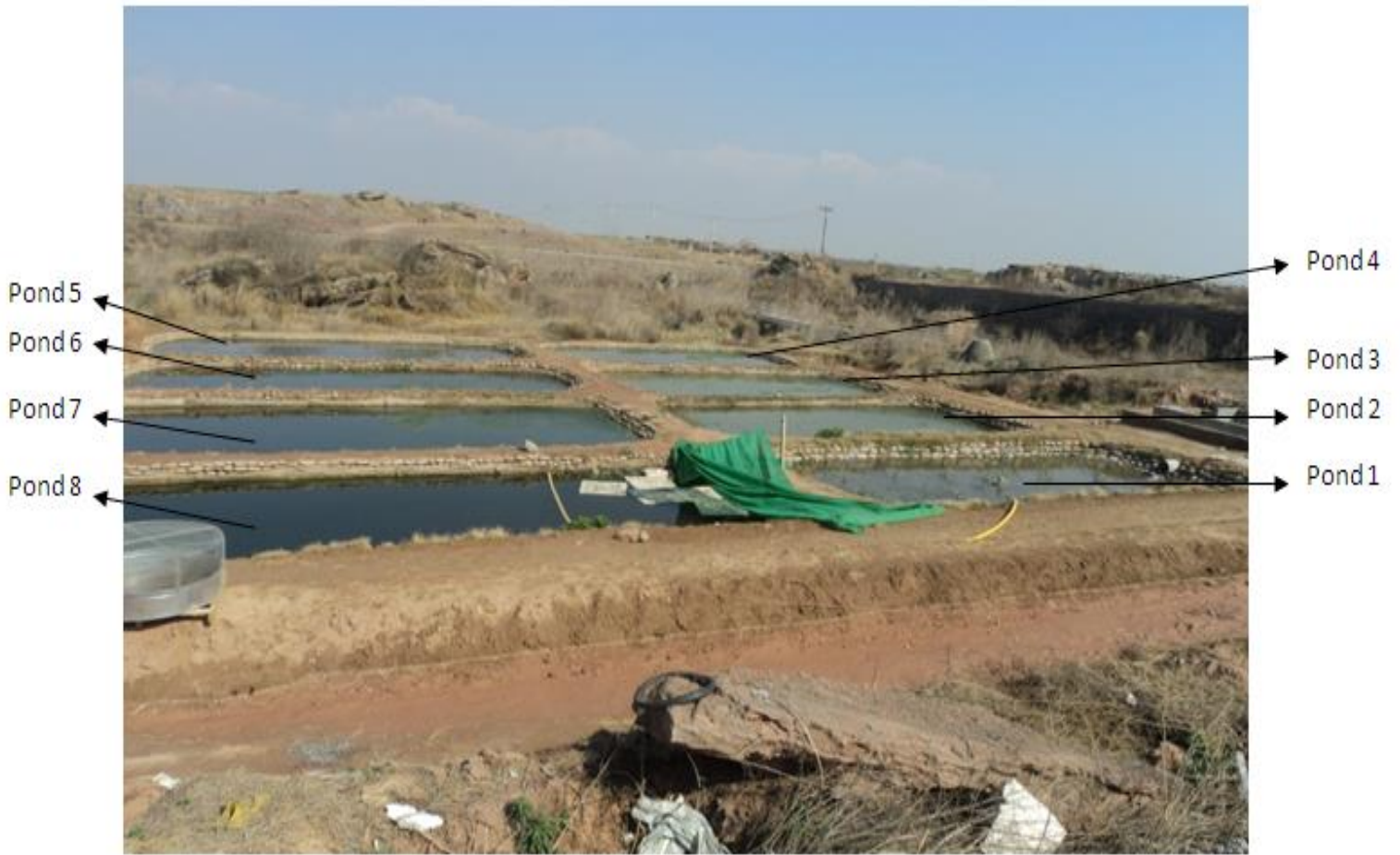
Fig 7: Pilot scale plant during construction phase
