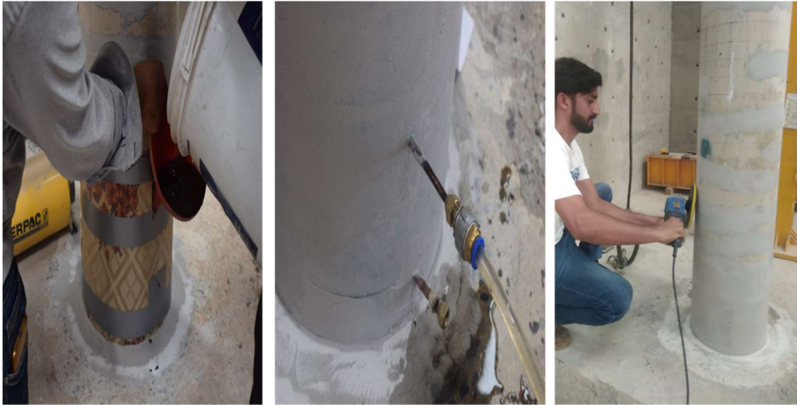
a) Application of Epoxy mortar (Sikadur 42) for patch works.
