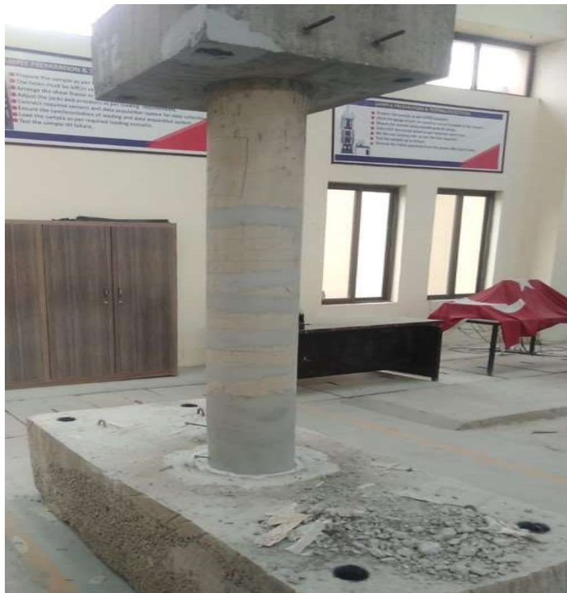
Figure 4.6: Repairing of column hinge concrete and reinforcement with sikadur epoxies.
