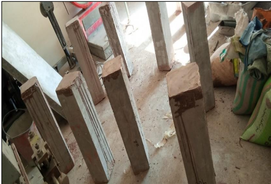
Figure 24: Sulphur capped all columns
