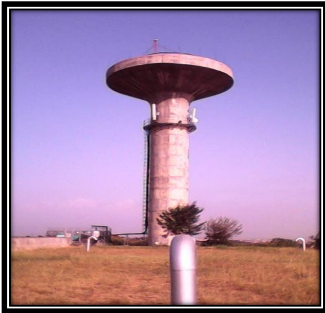
Over Head Tank (Gate 1)
