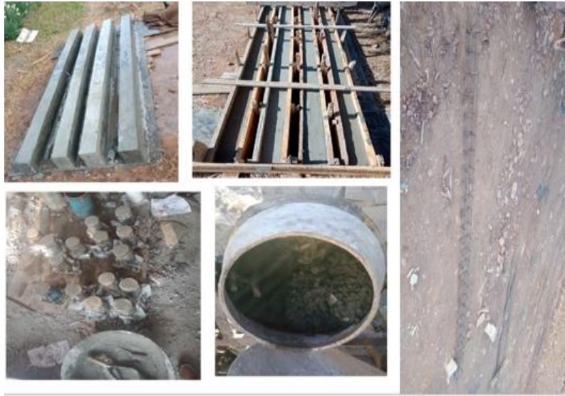
Figure 4.8 Casting of RCC Beams
