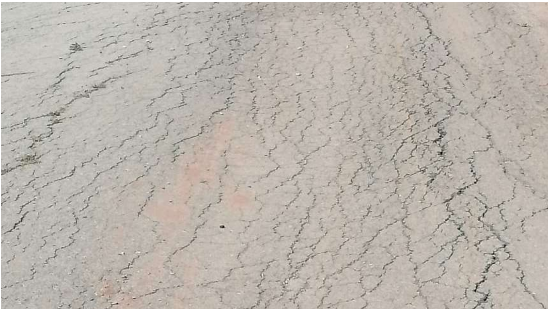
Figure 2 Rutting of road due to poor subgrade
