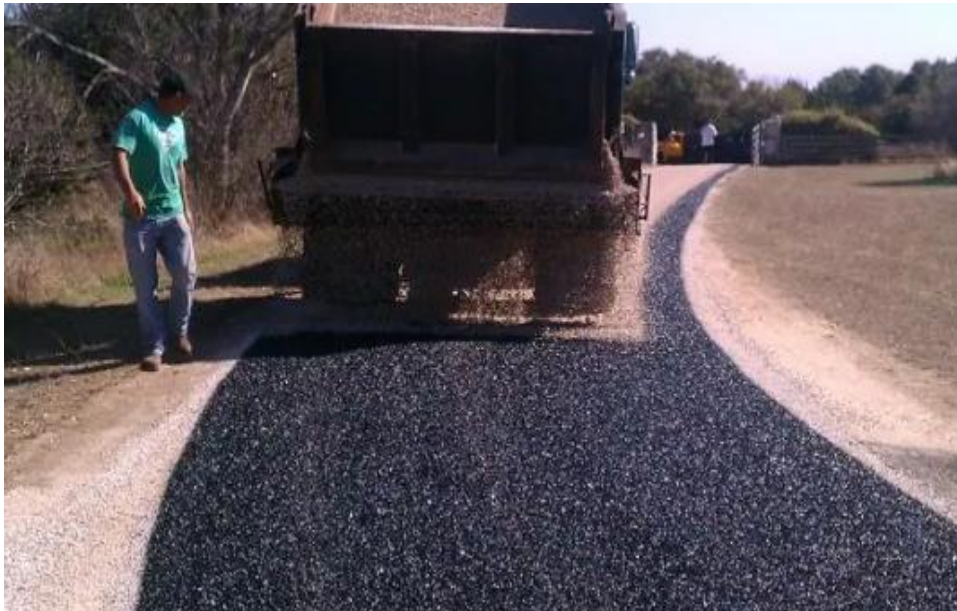
Figure 4. 4: Manually doing Chip Seal
