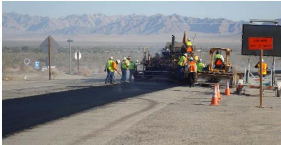
Figure 4. 5: Road during Overlay
