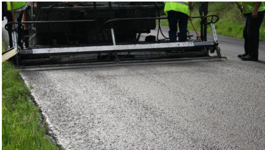
Figure 4. 1: Condition of Road During Micro Surfacing
