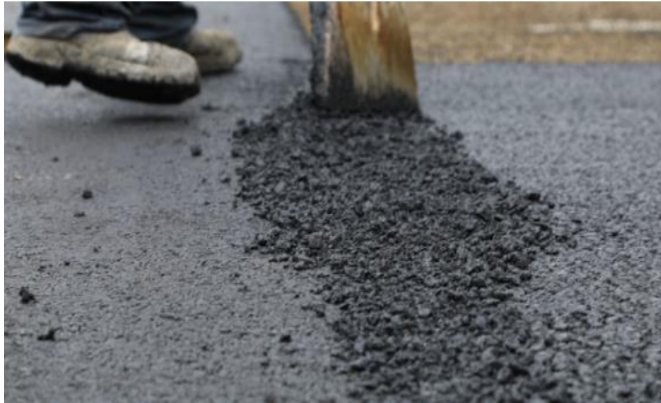
Figure 4. 3: Manually doing Chip Seal
