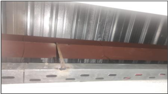
Figure 13 Beam under monitoring
