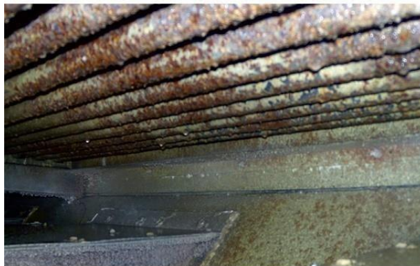
Figure 9: Water cooling towers
