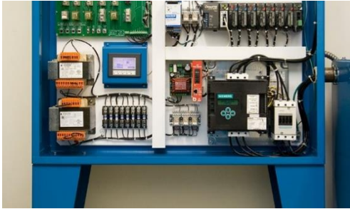
Figure 2: Elevator Controller
