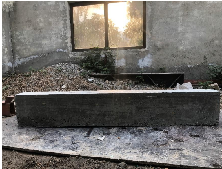
Fig. 6 feet long beam
