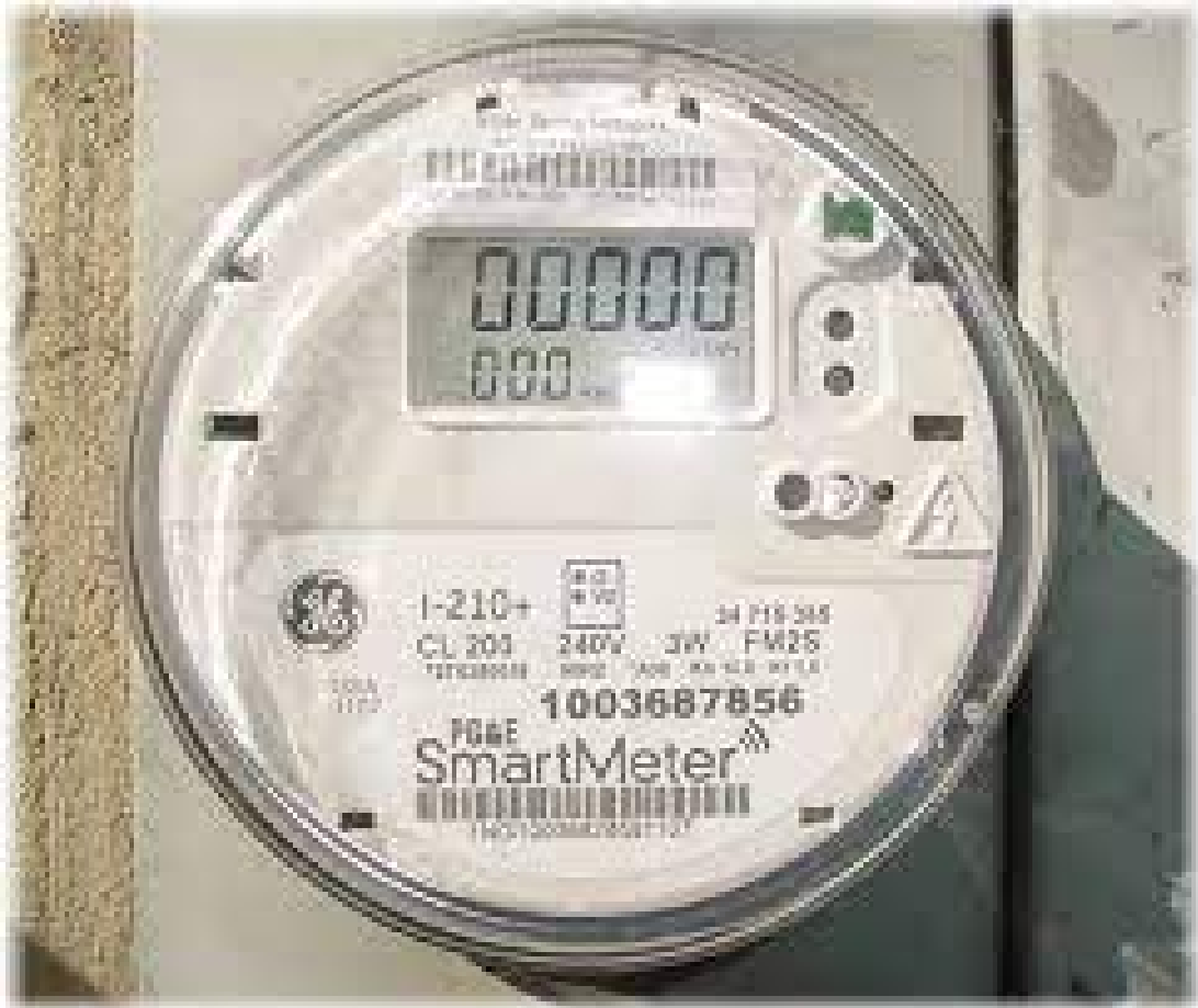
Figure 1.5: Smart Meter
