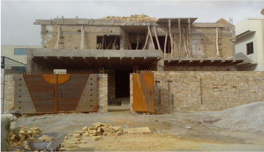
Figure 4.3: Un-Reinforced Brick Masonry- Cement Mortar (Structure type III), Source: field work
