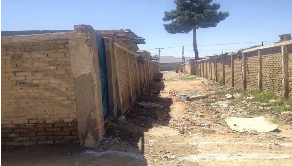
Figure 4.4: Un-Reinforced Brick Masonry- Mud Mortar (Structure type IV), Source: field work
