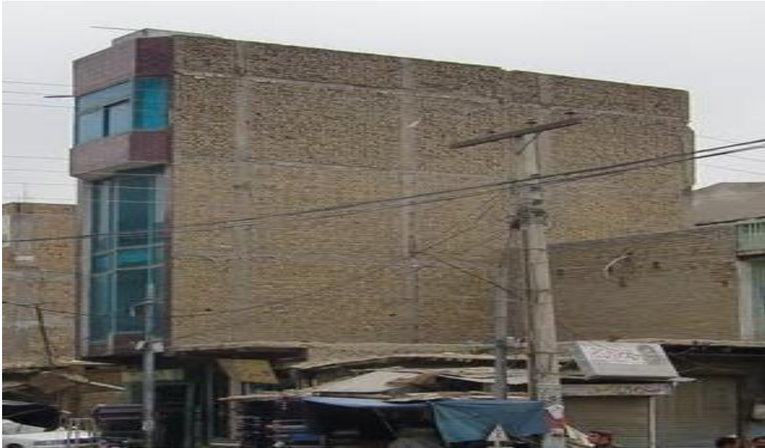
Figure 4.2: Reinforced Concrete Frame with infill masonry (Structure type II), Source: field work
