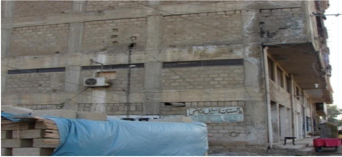
Figure 4.1: Reinforced Concrete Framed (Structure type I), Source : field work
