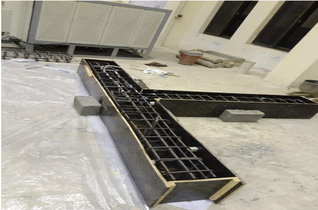
Figure 4.2. Casting of samples (a,b) Casting of Monolithically sample, (c) Formwork
