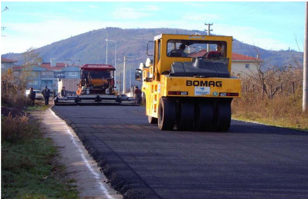
Figure 2.3 Asphalt wearing course being laid and compacted
