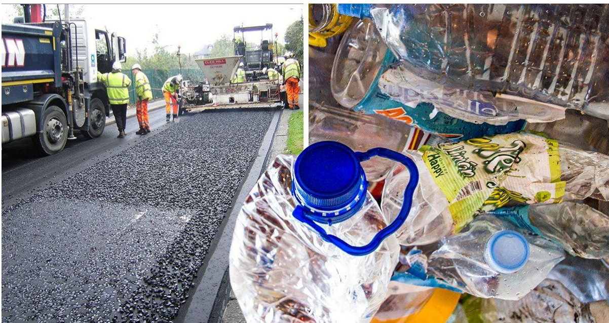
Figure 2.10 Plastic waste enabled Asphalt
