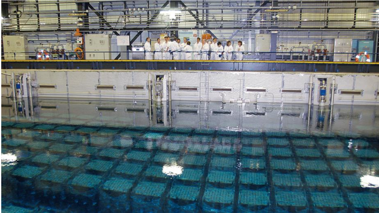
Figure 1.2 Spent nuclear fuel pool, copied from https://www.oecd-nea.org/jcms/pl_47481/spent-nuclear-fuel-pool?details=true .
