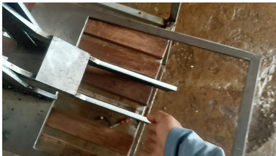
Figure 45 Welding of machine parts
