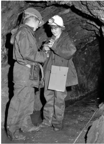
Figure 4.17 Students undertaking an underground geological mapping exercise at Dolaucothi gold mine, Mid-Wales. Note the tape measure laid out along the adit floor marking distances away from a mine survey point. Mine survey points are usually marked by bolts drilled into the adit roof.
