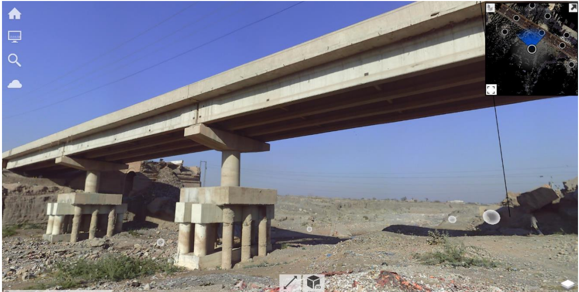
Figure 13 Snap of model obtained through TLS.
