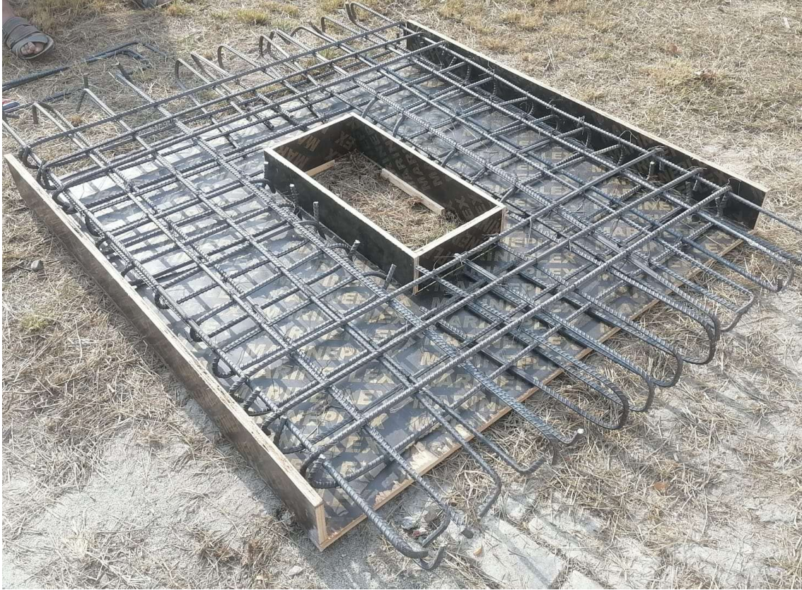
Figure 5: Web Reinforcement for Wall 1:2
