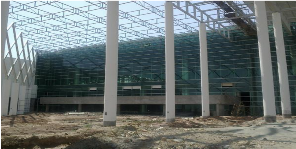
Figure 5.1 : Under construction view of terminal building
