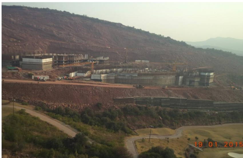
Figure 5. 6: Under construction view of Sheraton Hotel
