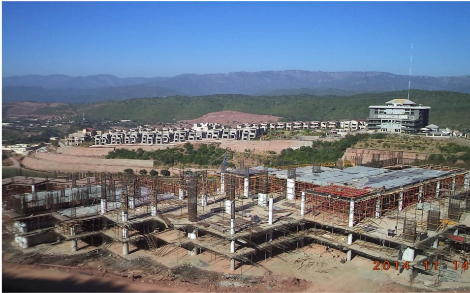
Figure 5. 7: Under construction view of Sheraton Hotel
