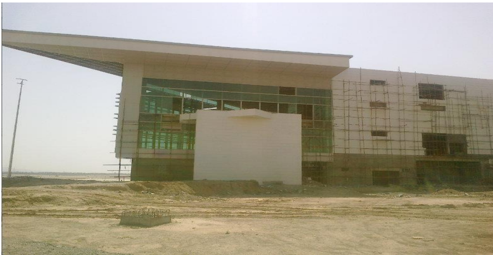
Figure 5.2: Under construction view of terminal building
